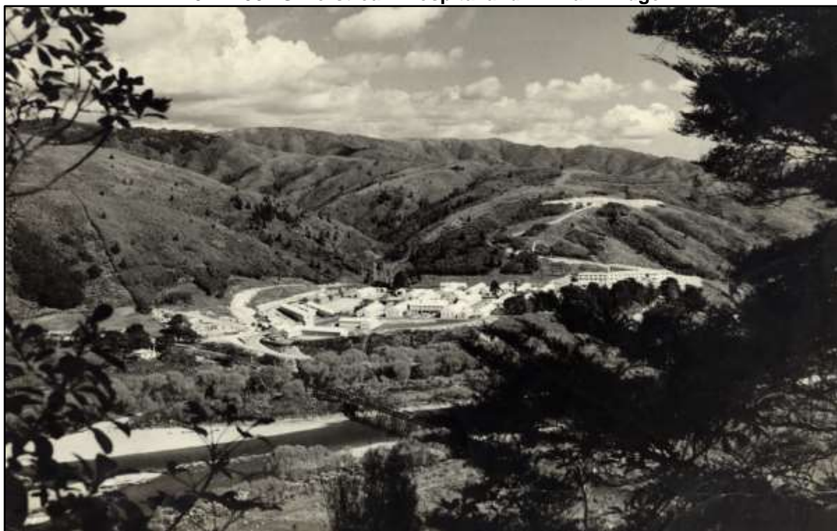
(Reference Upper Hutt City Library Heritage collection 1944-1954 Silverstream Hospital and 2 nd Rail Bridge)
