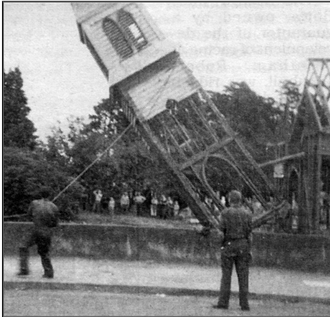
Pulling down St Joseph's Church Bell Tower
