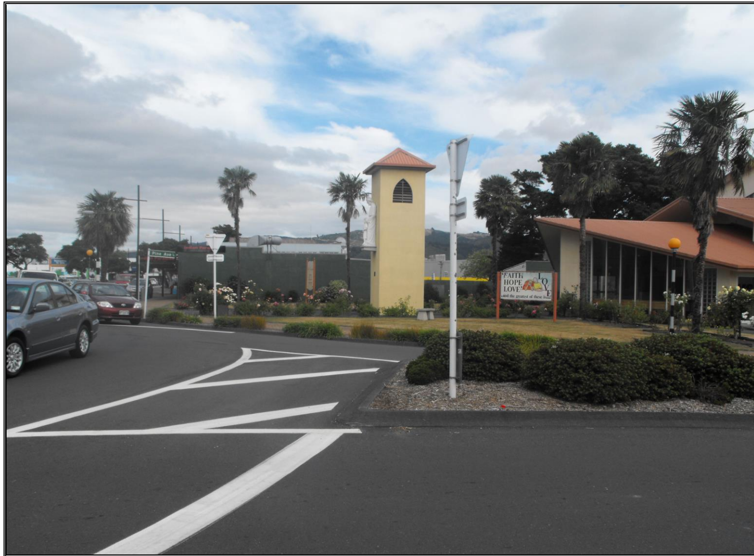
St Joseph's Church new Bell Tower
