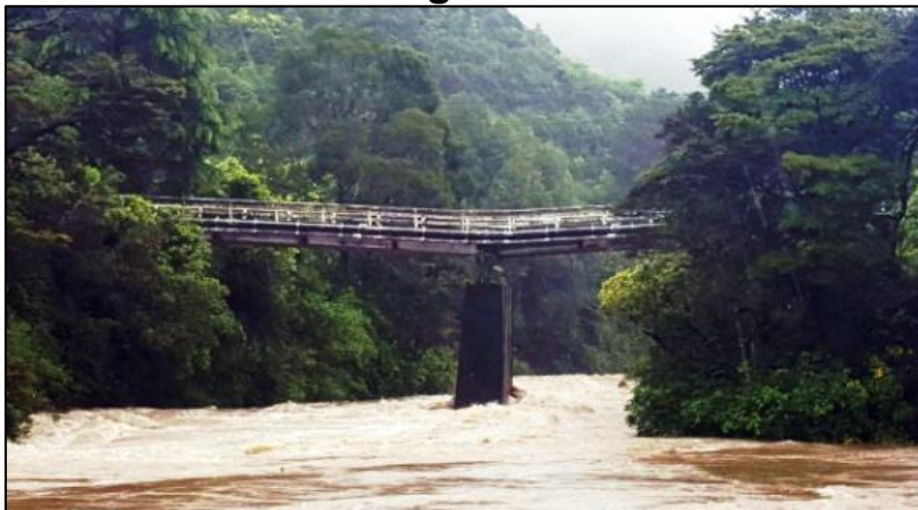
(Reference UH City Recollect website Akatarawa Bridge Tommy Livingston photo 29 Oct 2015)
