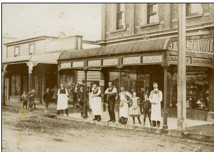
(Reference Upper Hutt City Library Heritage collection Recollect website 1906Hazelwood building P3-91-308)
