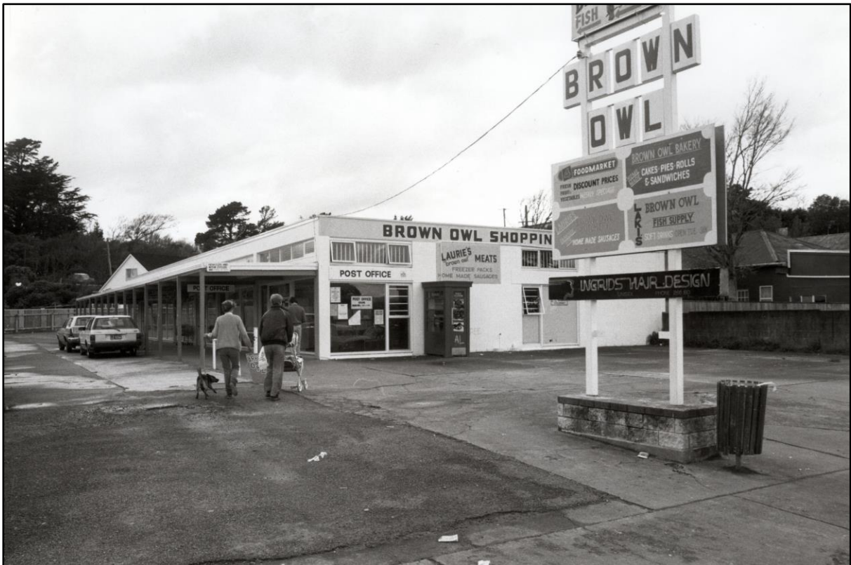
(Reference Upper Hutt City Library Heritage collection taken September 1984 UH Leader 02 October 1984)
